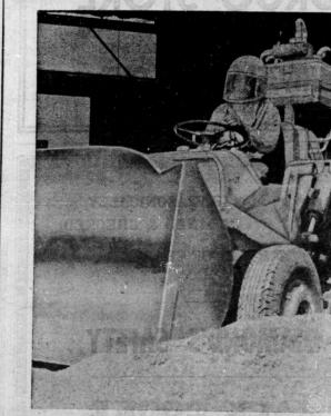
AIR-CONDITIONED — Space-age feed yard worker wears air-conditioned helmet while driving scoop shovel in Thermal, Calif., where the temperature sometimes soars to 120 degrees. With the helmet, workers are able to work continuously. Previously, heat forced them to rest at frequent intervals. Thermal often is the U.S nation's hottest city.
