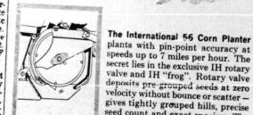
plants with pin-point accuracy at speeds up to 7 miles per hour. The secret lies in the exclusive IH rotary valve and IH "frog". Rotary valve denosits predenosits pre-grouped seeds at zero velocity without bounce or scatter — gives tightly grouped hills, precise seed count and exact spacing. The "frog" forms and firms the seed zone – for even depth and uniform
