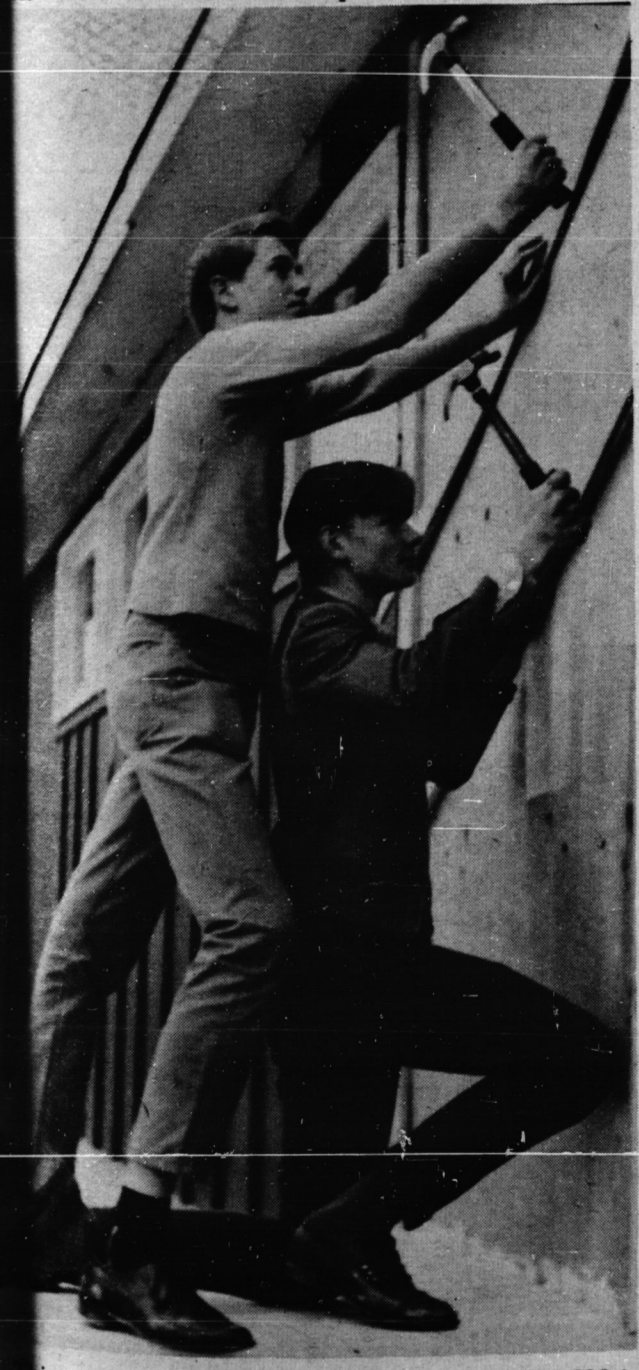
This portable classroom costing an estimated $3,500 is to be put in use at the Hagersville Secondary School. By Reitsma, (left) 16, of R.R. 3, Caledonia, and Elgersman, 16, of R.R. 1, Caledonia, do their part project. (Photo by James Mercer)
