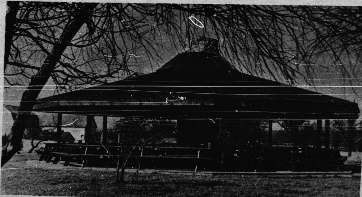
This pavilion is part of the facilities at the Haldimand County Park, which the council decided to return instead of turning it over to the Big Creek Region Conservation Authority. (Record Photo)
