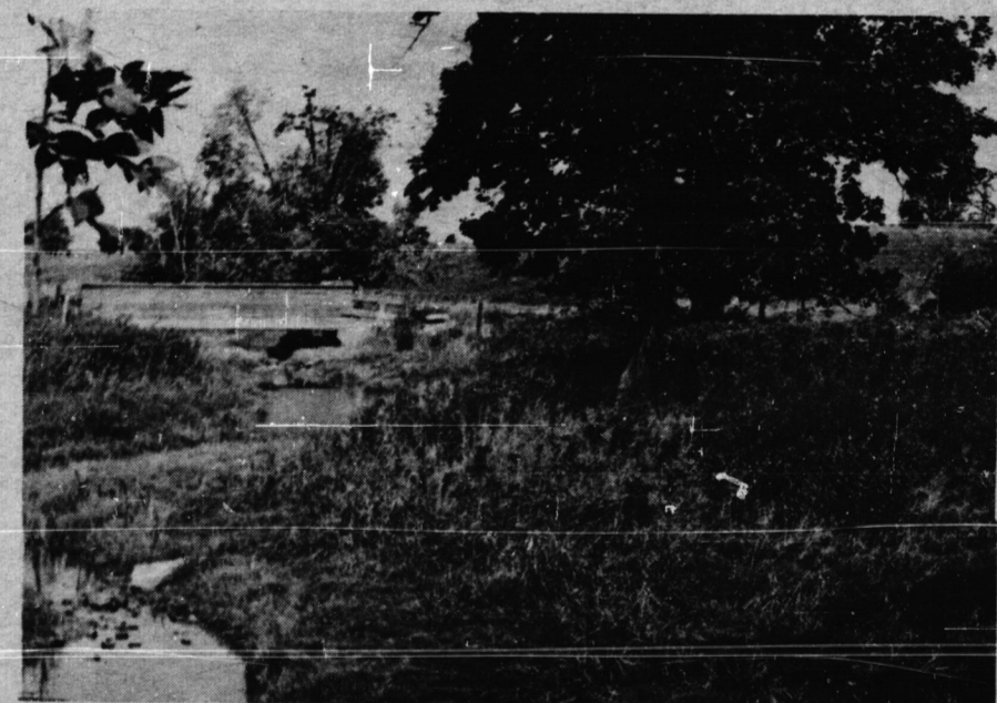
This bridge spanned regular creek. (Photos by Jim Mercer)
