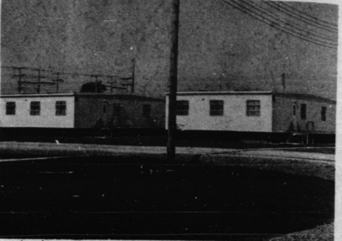
At the peak of construction in 1971, the work force is expected to reach 1500 men at Ontario Hydro's Nanticoke plant. This camp will accommodate up to 2000 employees at the site. A common kitchen will be used to feed the workers. (Staff Photo)
