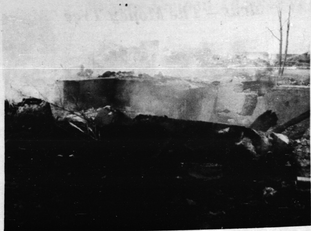
Debris and smoke is all that's left of a former house on the Texaco site. Cohen and Cohen of Ottawa has the contract for the clean up job. (Staff Photo)
