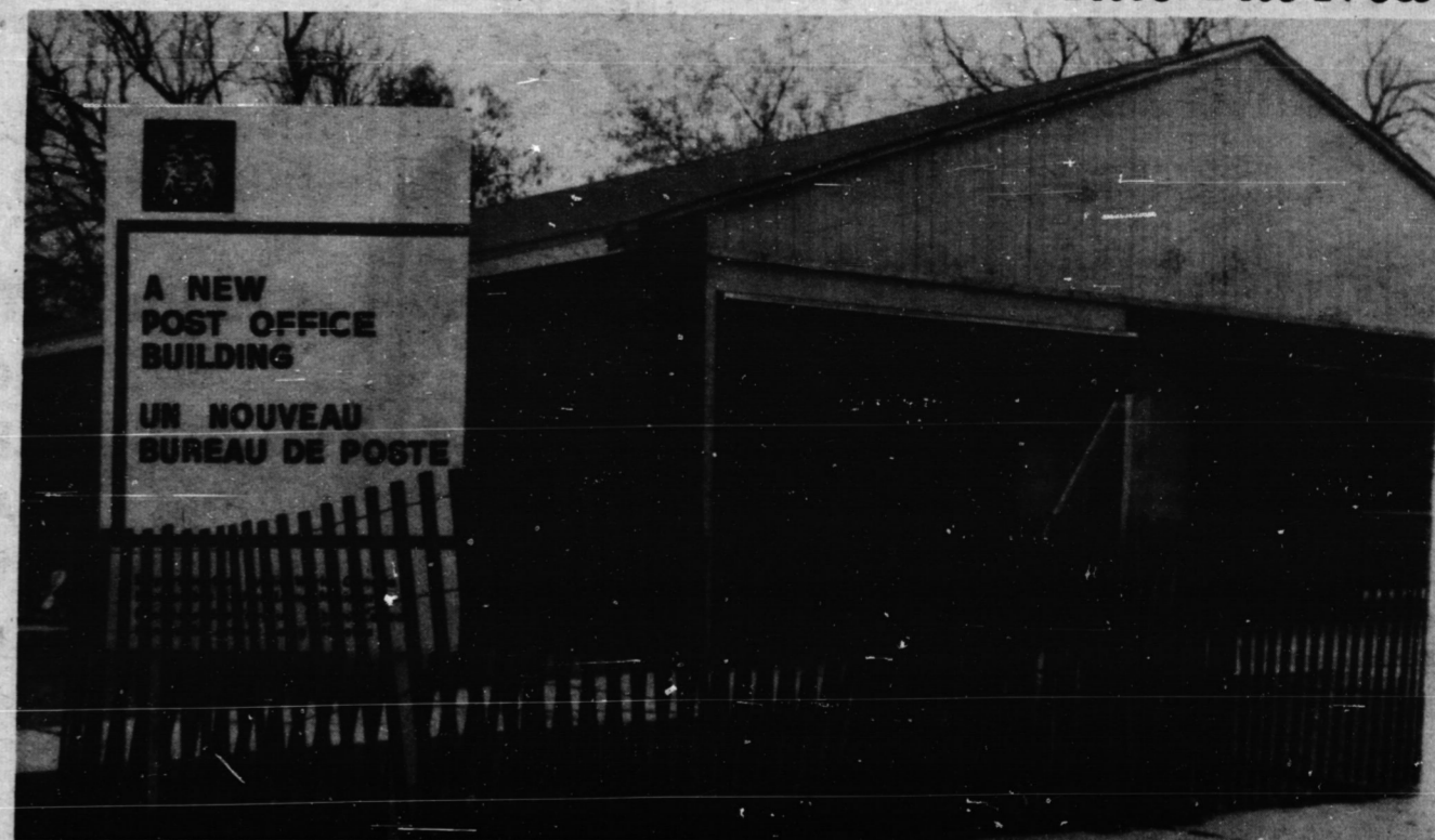
Cayuga has a new post office which was occupied by the employees Monday. (Staff Photo)
