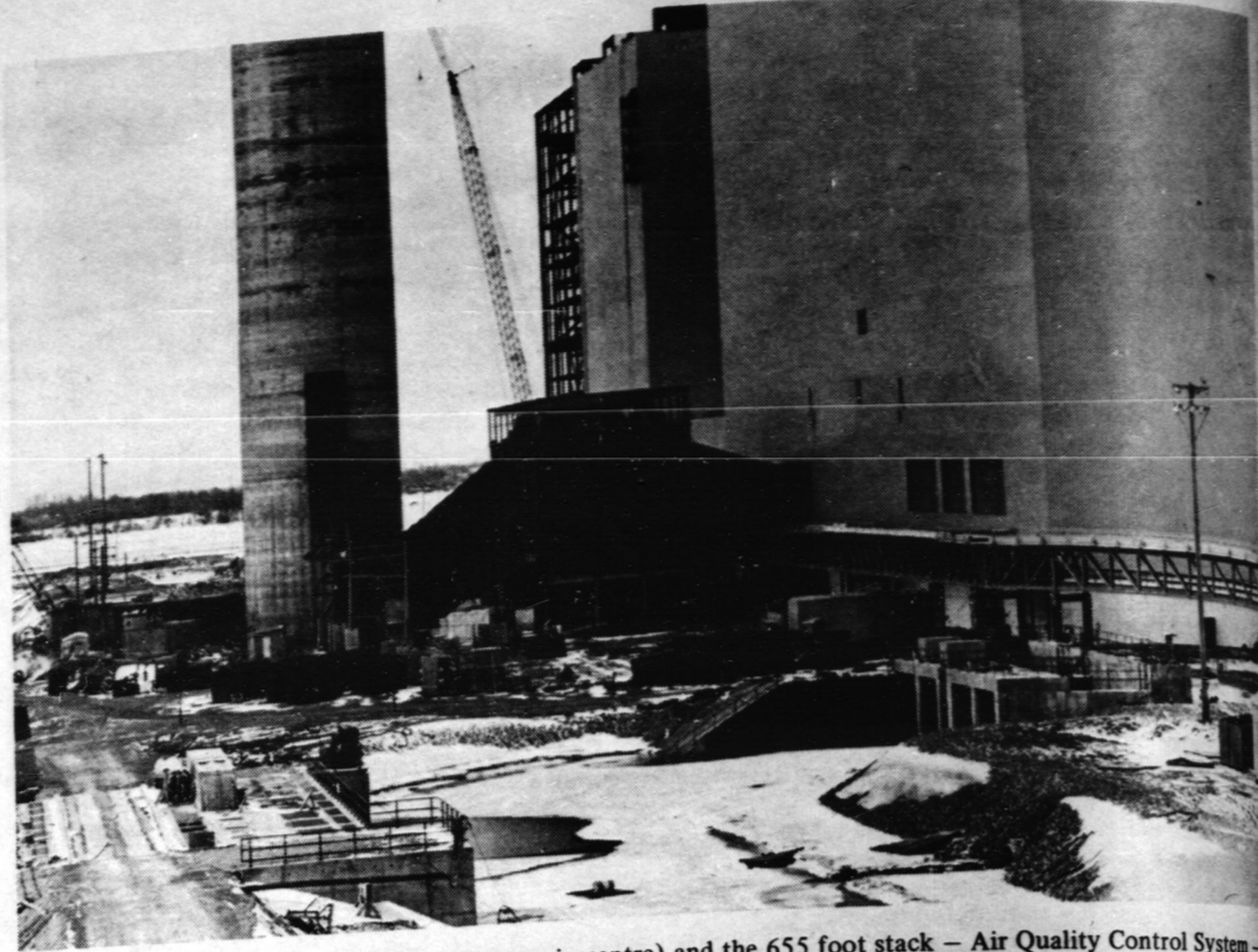
The Electrostatic Precipitator (box-like structure in centre) and the 655 foot stack - Air Quality Control System - will be utilized for the first time when the first Nanticoke G. S. boiler system is "smoke-tested" on May 14.
