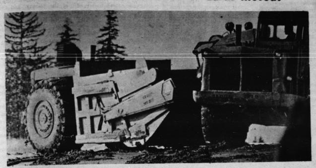
mover with a capacity of 32 cubic yards of earth. Weighing 49 tons empty and approximately 100
