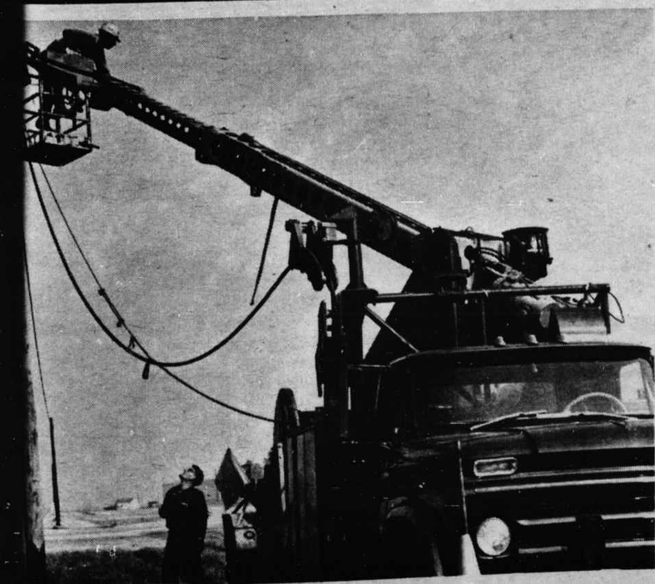
Bill Bigham, of Woodstock, works up in the bucket of this Bell Canada truck as the Sandy McRae, of Simcoe, string 50-pair telephone cable at the International Plowing Match site near Jarvis. When they complete their work, almost two miles of cable will have been placed in readiness for the event. (Staff Photo)
