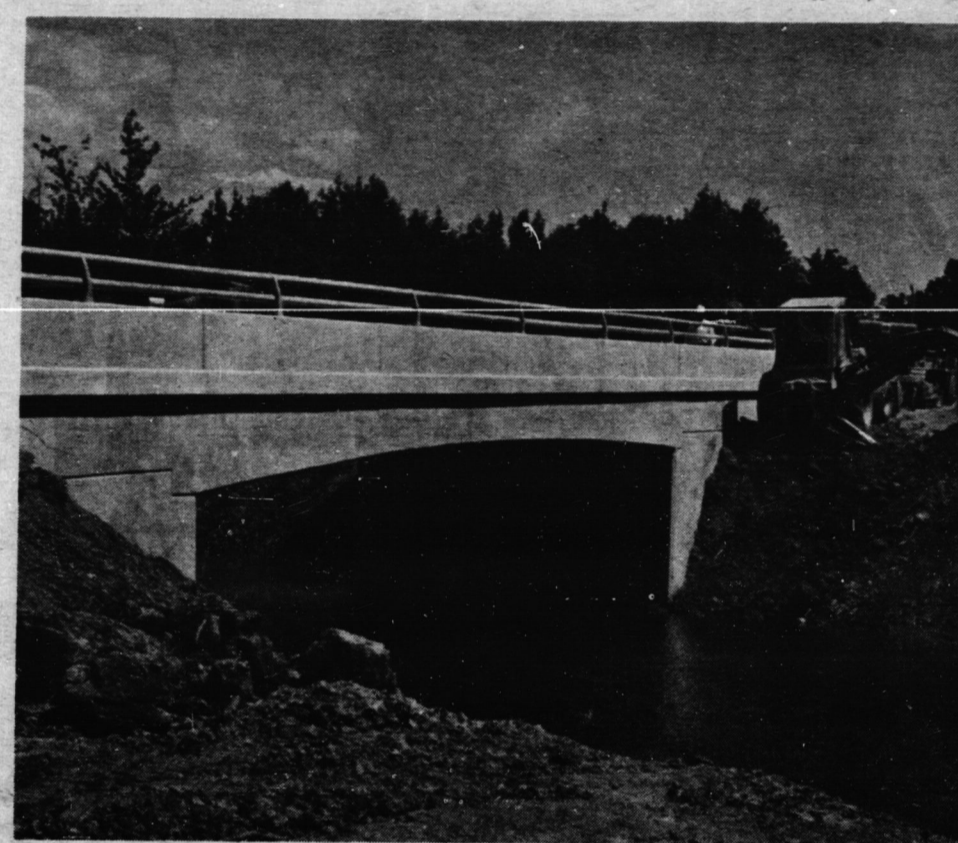
With the exception of finishing touches, work on the new $49,130 Reicheld Bridge over the Sandusk Creek on Conc. 4 Walpole Township, is all but complete. (Staff Photo)
