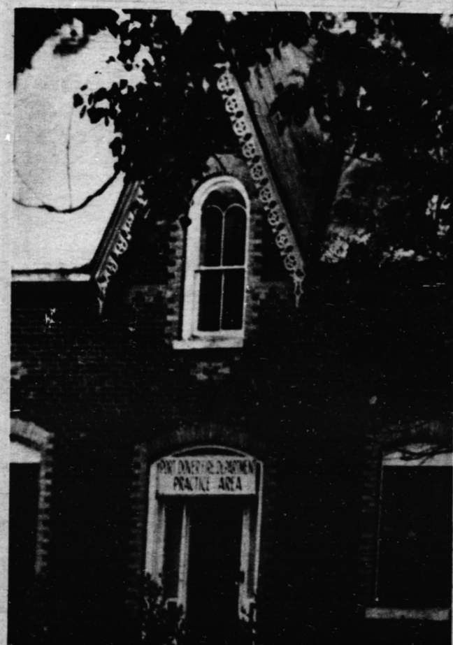
An abandoned farm house on Stelco property on the Norfolk-Haldimand boundary is being used as a practice area by the Port Dover Fire Department. (Staff Photo)
