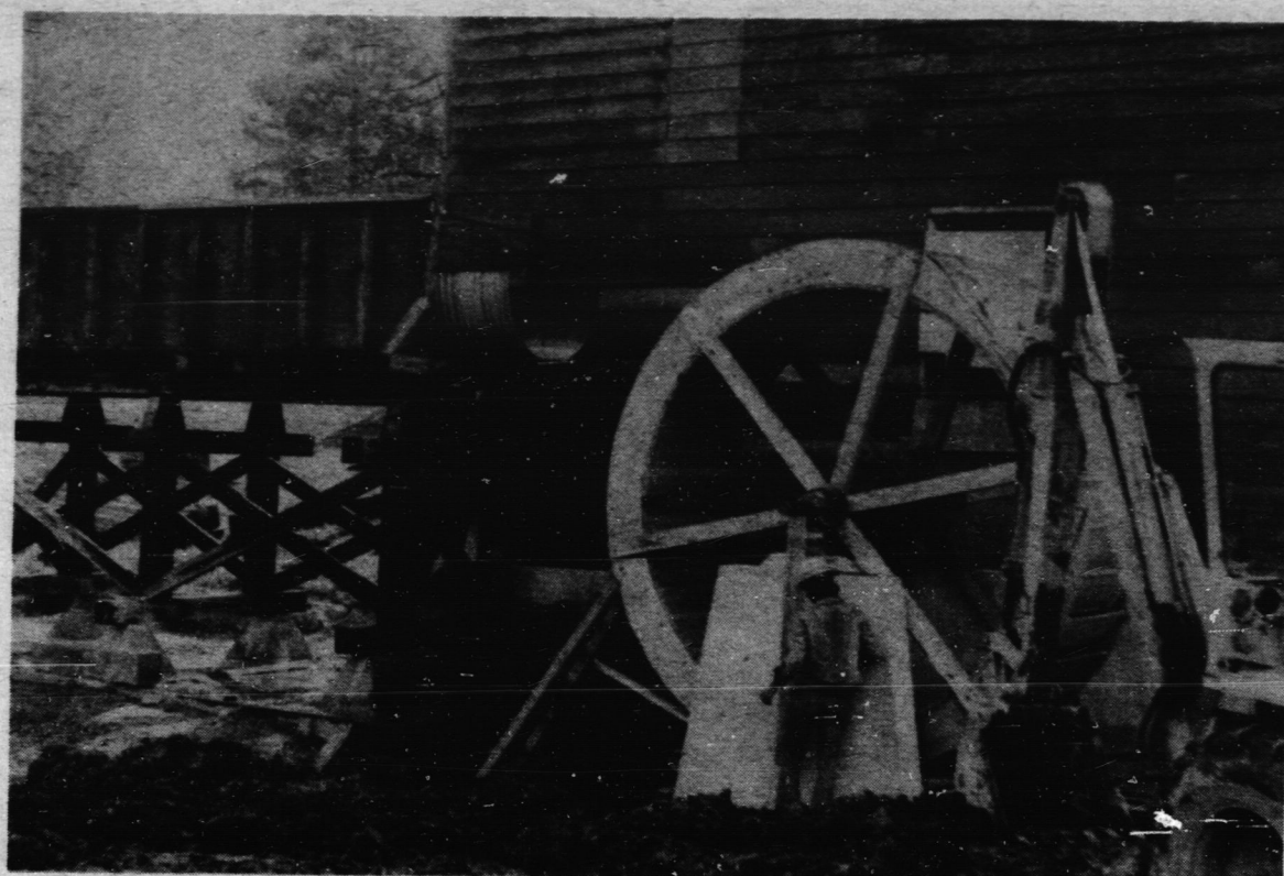
Workers at the Backus Mill secure the large overshot wheel in front of the flume. The mill should be operational before long as they are still waiting for a few parts. (Photo by Richard Houghton)
